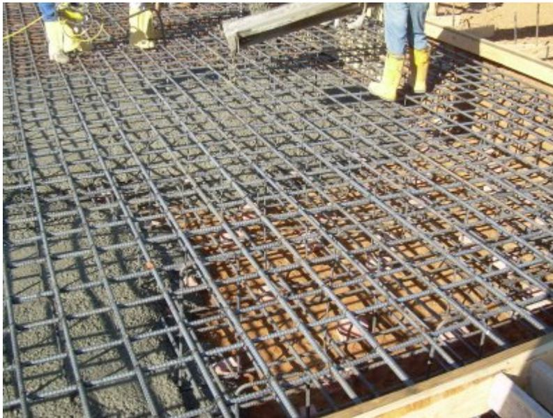
*Pouring concrete into the tower foundation.*
